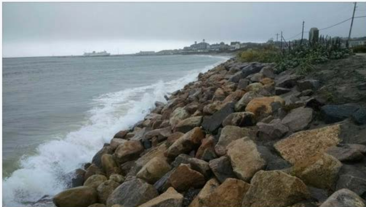
"Corn Neck Road revetment"
